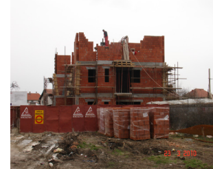
Velika Plana - construction site, social housing in protected environment, March 2010.
