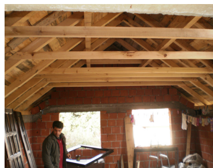
Grocka – construction material installation, February 2010.
