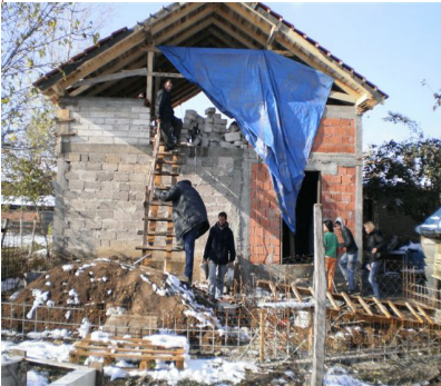
Mladenovac, DRC field visit, construction material installation, November 2009.
